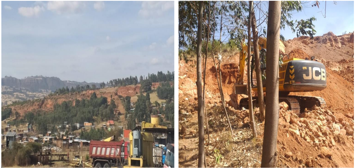
Figure 3. 4: Ambo sandstone mountain (Left: Senkele Mountain, Right: Excavation of the sand)
