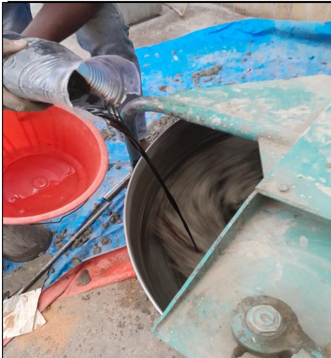
Fig. 5: Concrete mixing in horizontally rotating mixer
