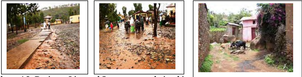
Photo 4.8: Drainage Line and Storm water relationship
