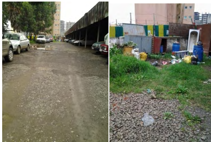
Figure 3- 64 Back yard of the building
