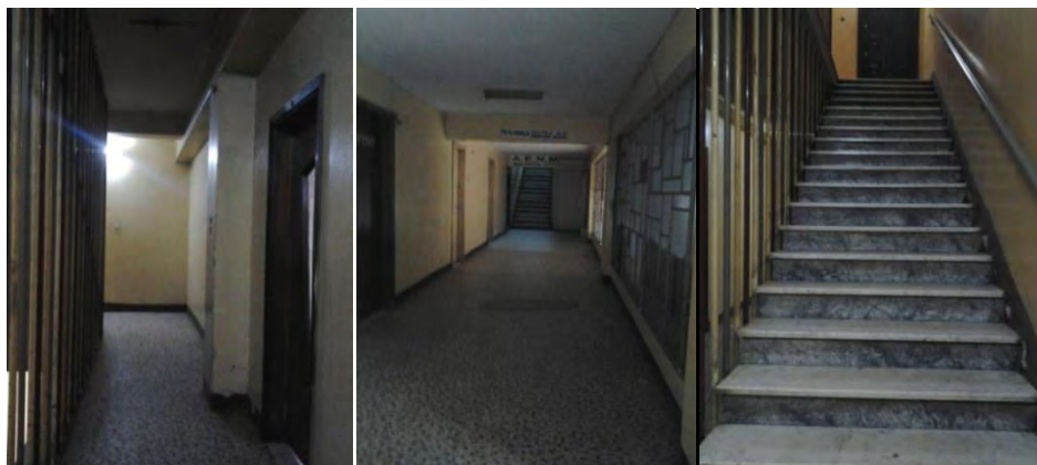
Figure 3- 12 Window and light in stairs and corridors
