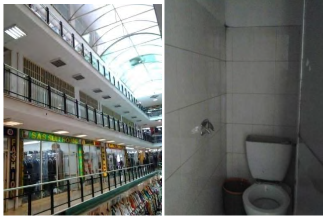
Figure 3- 49 Interior space of the building, sky light and toilet (from left to right)
