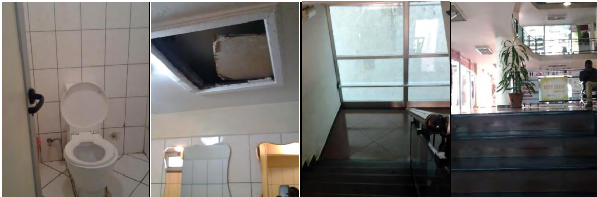
Figure 3- 53 Toilets in the building stair case and open down windows
