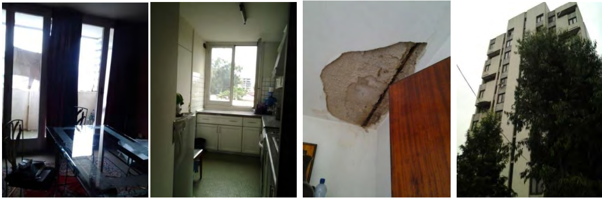
Figure 3- 65 Interior space of the apartment building
