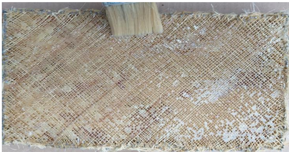
Fig. 12 impregnating woven sisal fiber with unsaturated polyester resin
