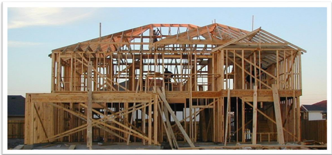
Figure 2-3: Wood frame houses under the construction (source Jaksmata, 2008 )
