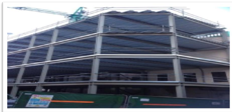
Figure 4-14: Composite steel decking constructions in London (decking supplies limited,2008)
