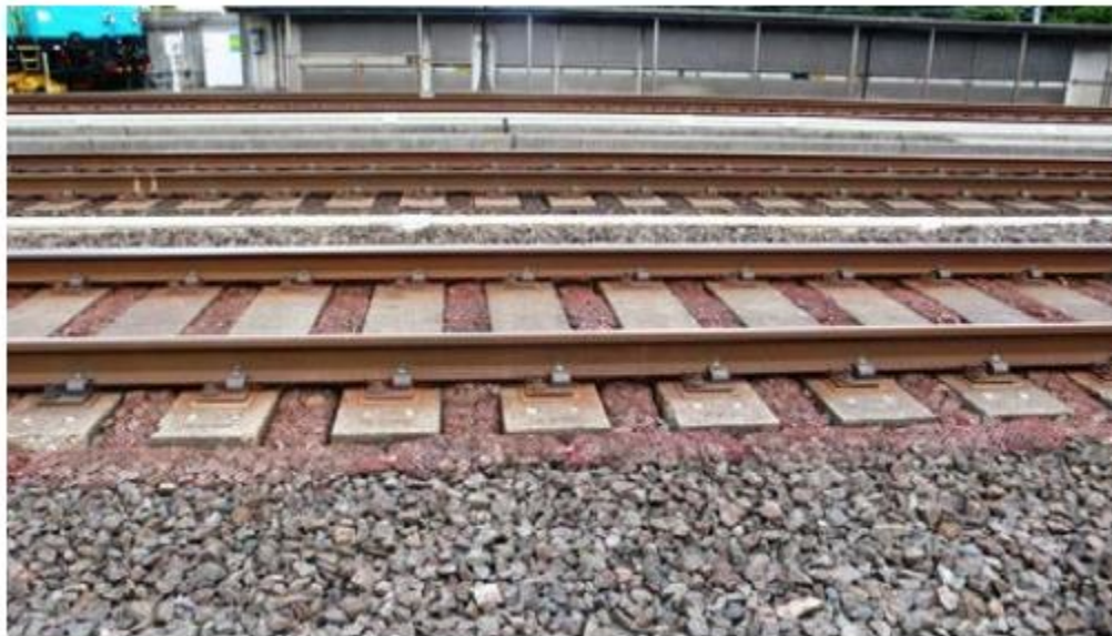
Figure 2.9: Ballast bags placed on the Japanese Shinkansen [1]
