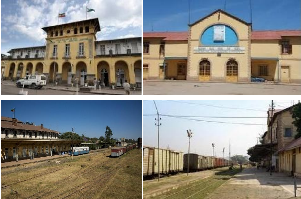
Figure 2.11: old railway station Addis Ababa and Dire Dawa [54]
