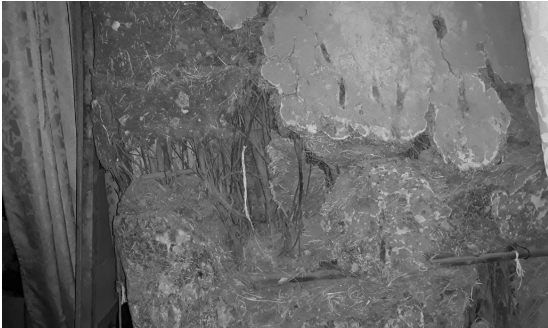
Photo: XIV The material that the church is built with and the kneeling down of the church
