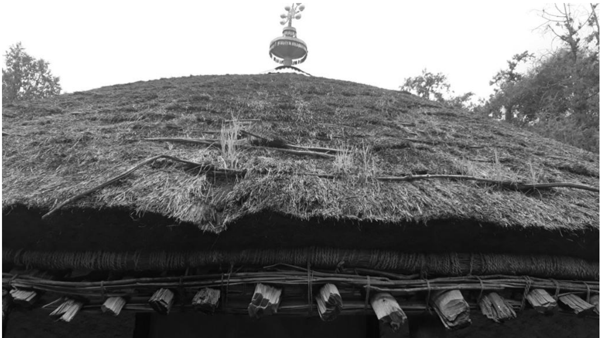
Photo: VIII. The roof of the Church
