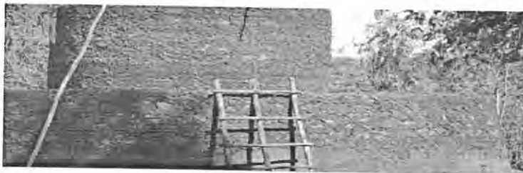
Fig 3.7: Esate kela, traditional house at Zege, (source: Abraham Marye et al., 2011)
