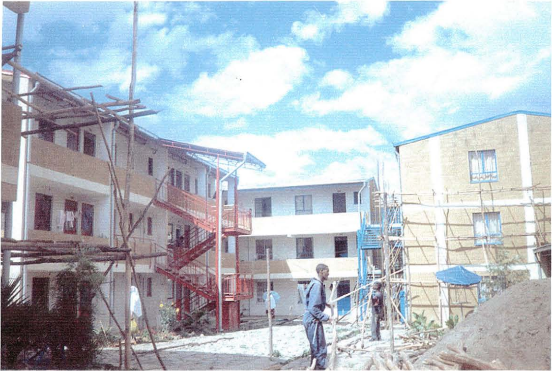
Figure 3.5: External wall plastering works in Kebena site. Photo taken from Kebena site.
