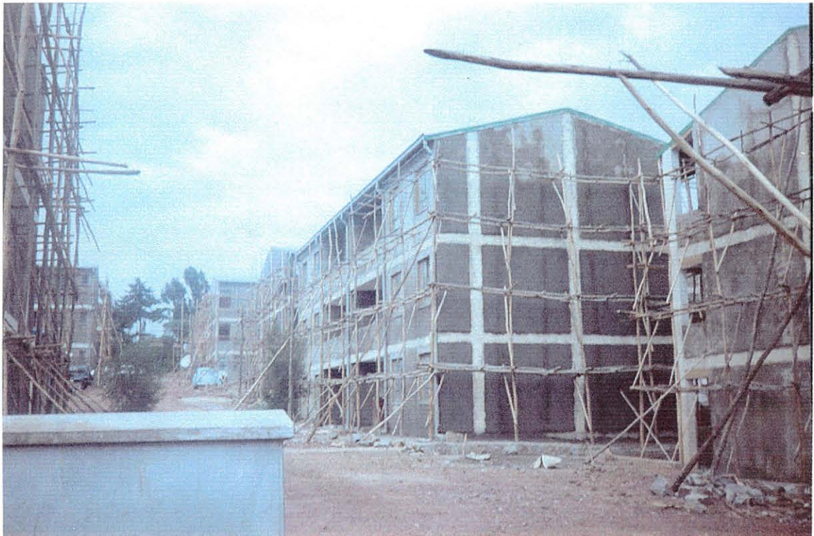
Figure 3.6: Plastered housing walls. Photo taken from Gulele I site.
