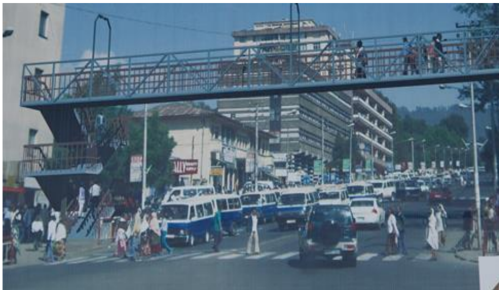
Figure 1.2: steel bridge for pedestrian around Arat killo
