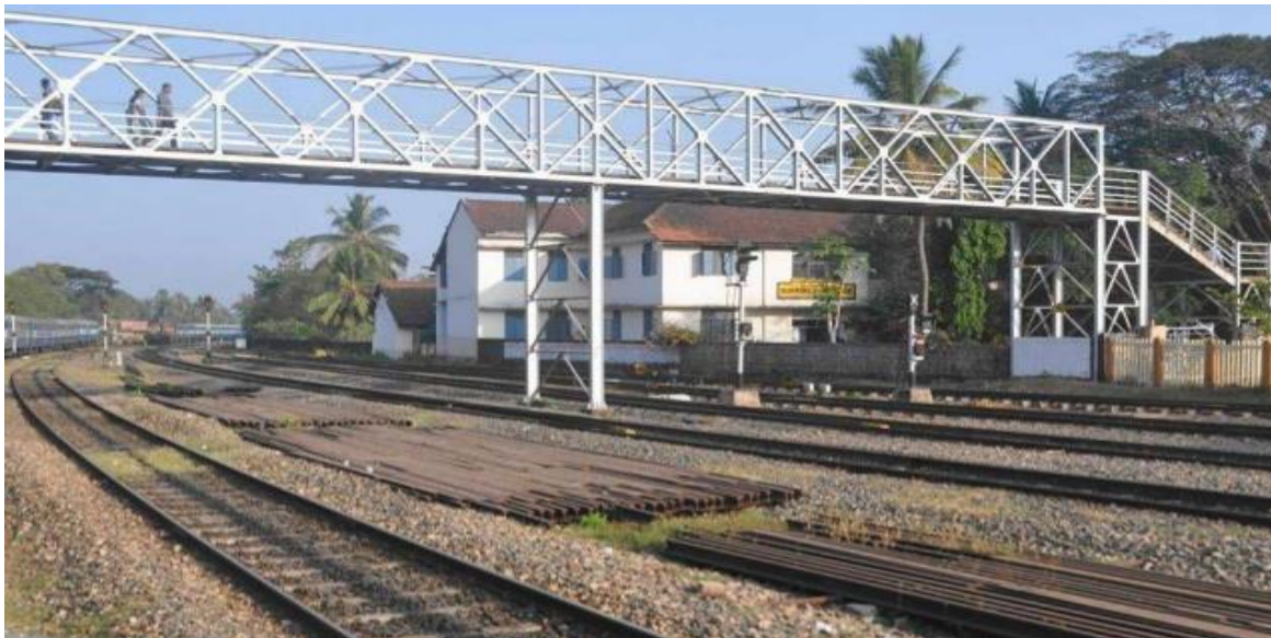
Figure 2.1: pedestrian steel truss bridge for crossing railway track
