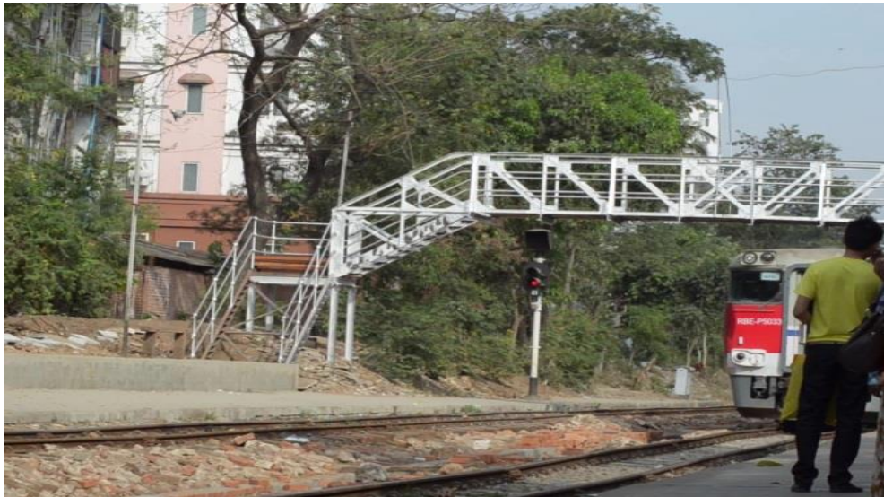
Figure 1.1: Train passing under pedestrian truss bridge
