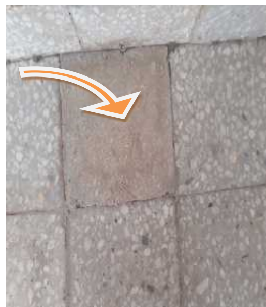
d) Different type of terrazzo tile is executed
