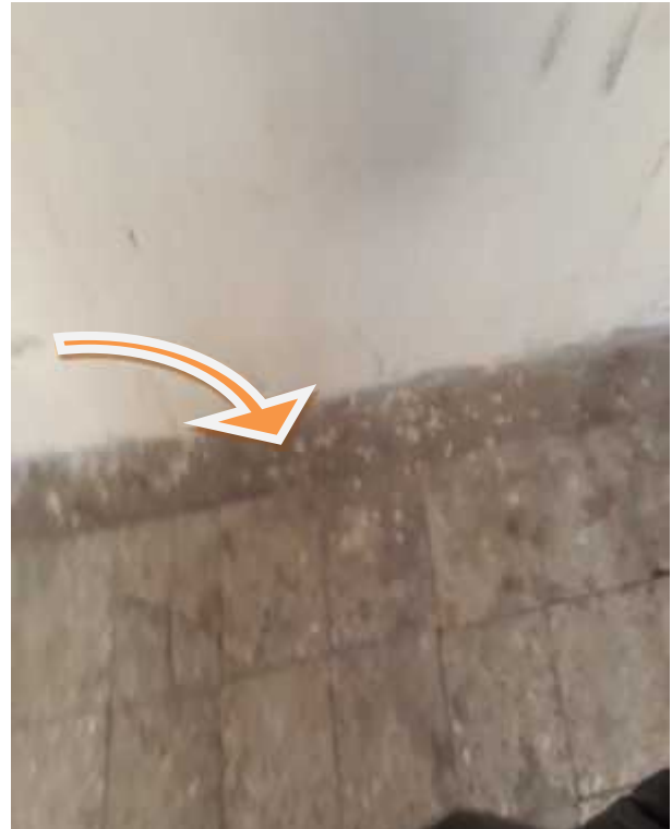
a) Cured mortar on terrazzo tile b) The gap b/n terrazzo tile & wall filled by mortar
