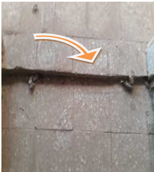
c) Level difference in floor
