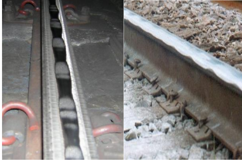
Figure 3.8: Rail roughness [9]
