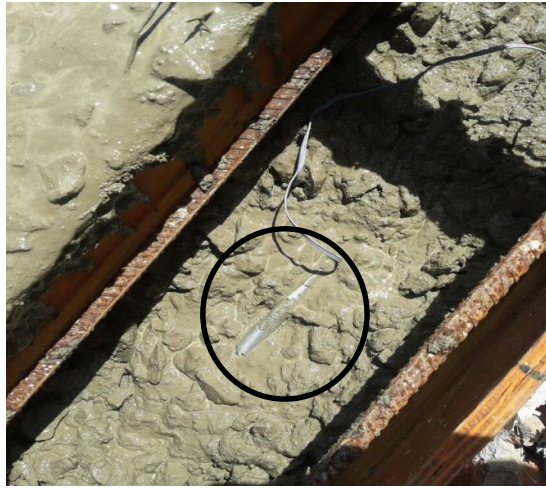
Figure 3-52 Placing of the mold strain gage
