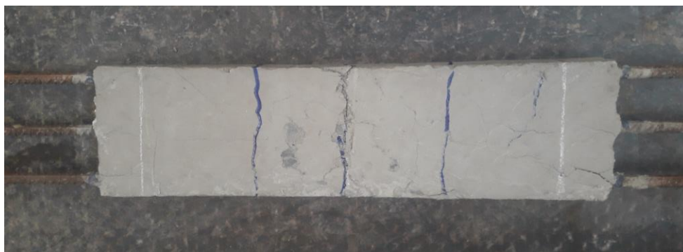
Figure 3-21 Cracks formed after trial damaged concrete section loading
