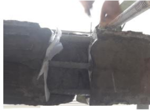
Bottom side of beam
