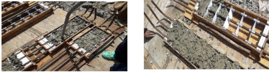
Figure 3-44 Casting of the damaged bond concert sections
