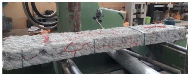
Figure 3-33 Trial beam damaged concrete section with roughened surface
