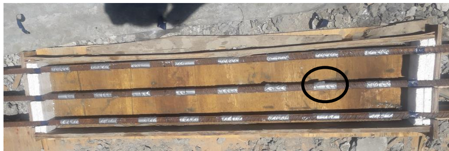
Figure 3-41 laminated paper used for slit formation
