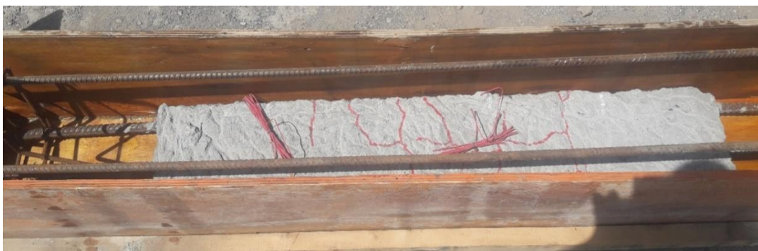
Figure 3-36 Placing of the top bars to the damaged concrete section
