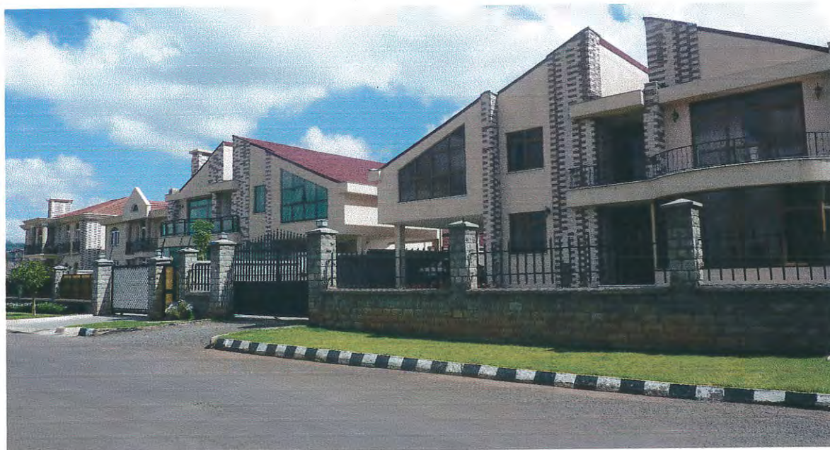
Figure 4.12: Sunshine Real Estate Villa type Houses at Meri Luke Site
