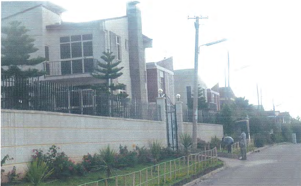
Figure 4.8: Ayat Real Estate G+1 Villa Type of Houses at Ayat Site
