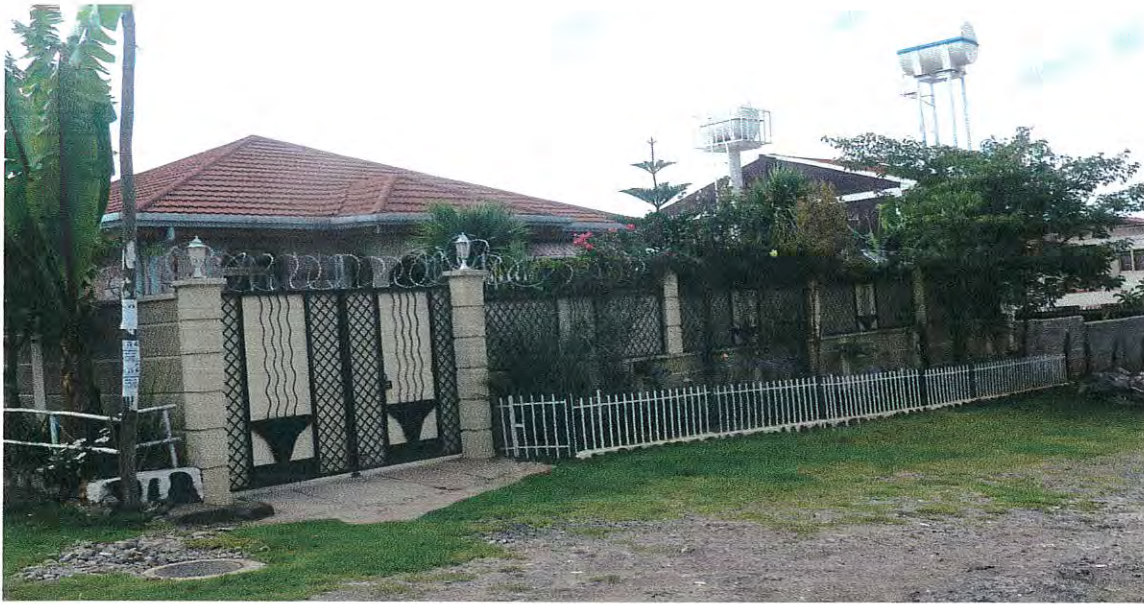
Figure 4.9: Ayat Real Estate G+0 Villa Type of Houses at Ayat Site
