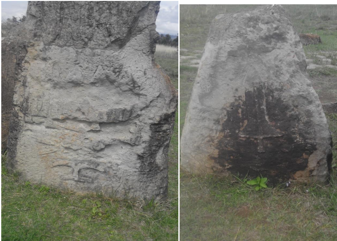
Figure 12: Deteriorating in structural conditions due to climate
