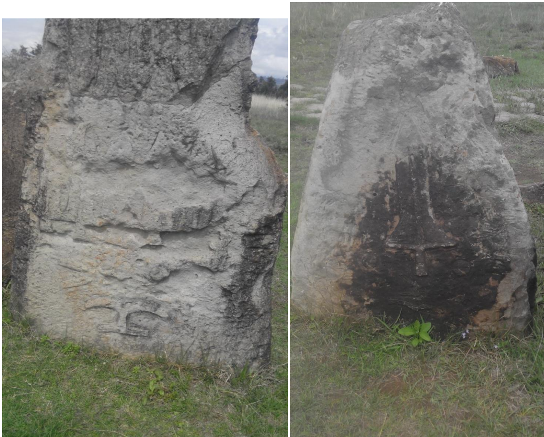
Figure 10: Deteriorating in structural conditions at Tiya WHS
