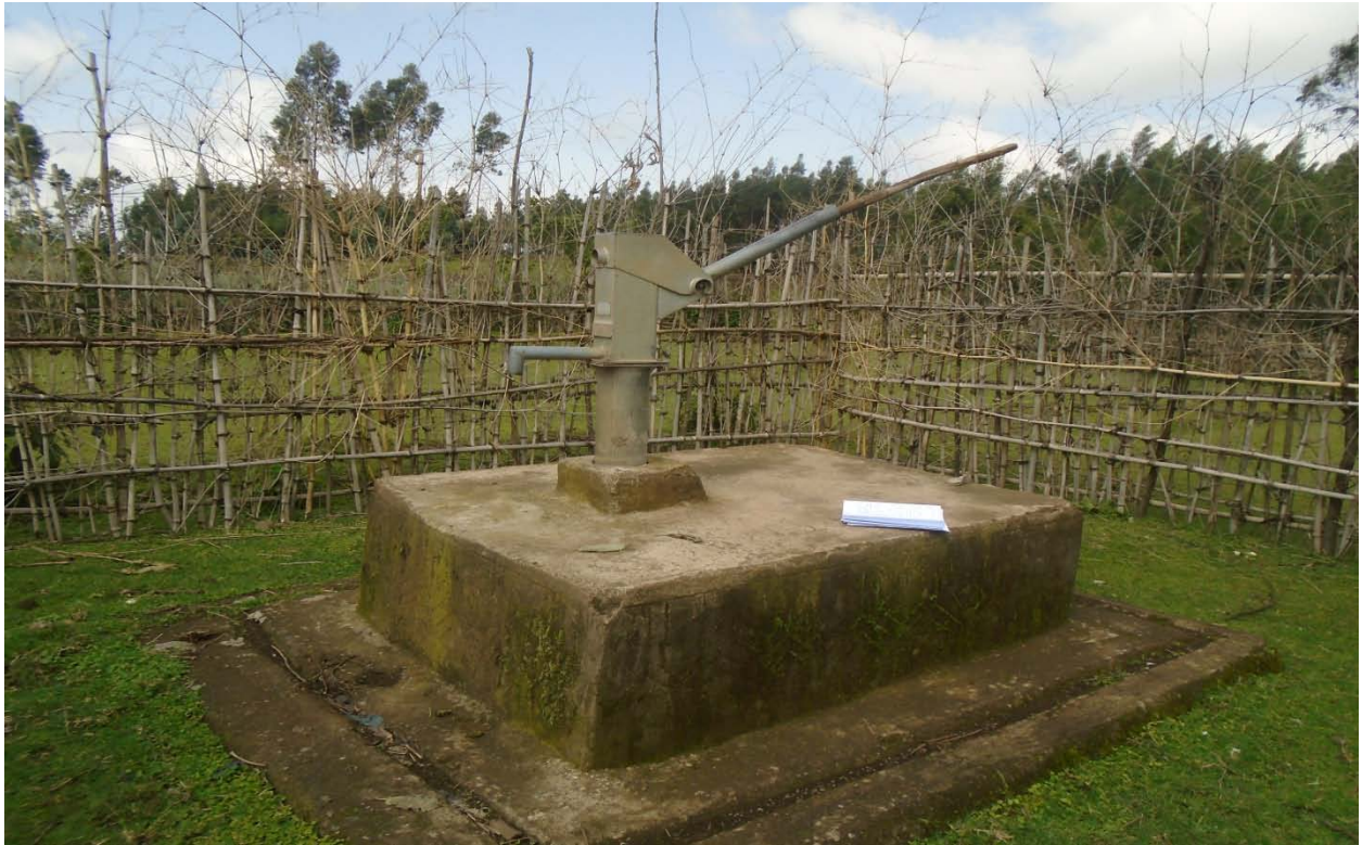
Figure 2 The hand pump used by the local community
