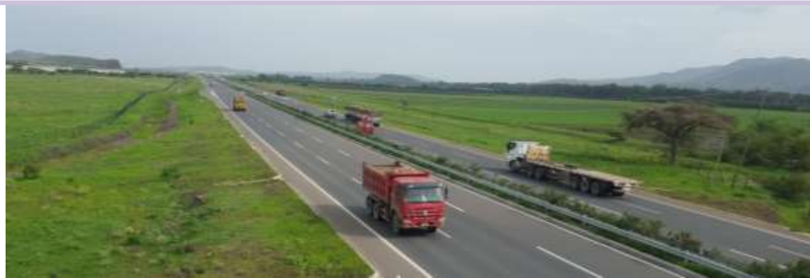
Picture at Chainage K26 + 650
