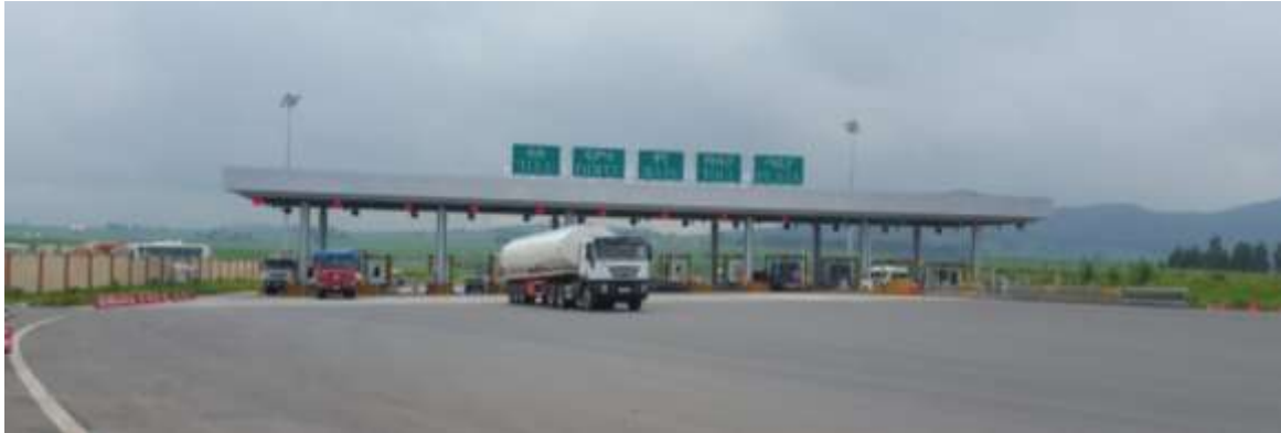
Addis Ababa – Adama Expressway Entrance Gate at Tulu Dimtu Main Toll
