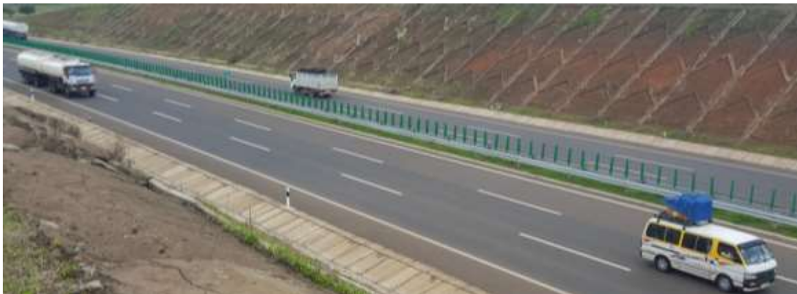
Picture at Chainage K56 + 070
