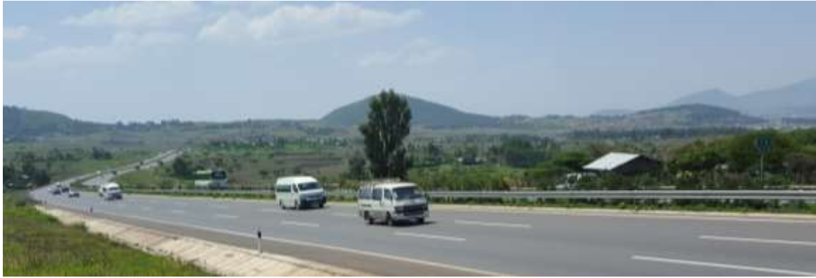
Picture at Chainage K9 + 990
