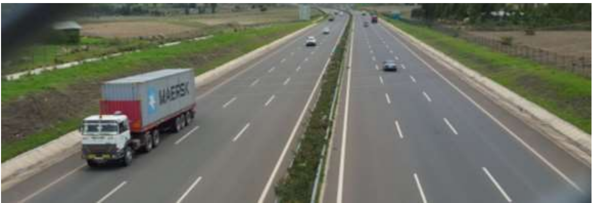
Picture at Chainage K4 + 050
