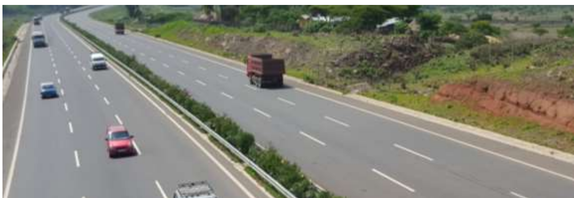
Picture at Chainage K9 + 660
