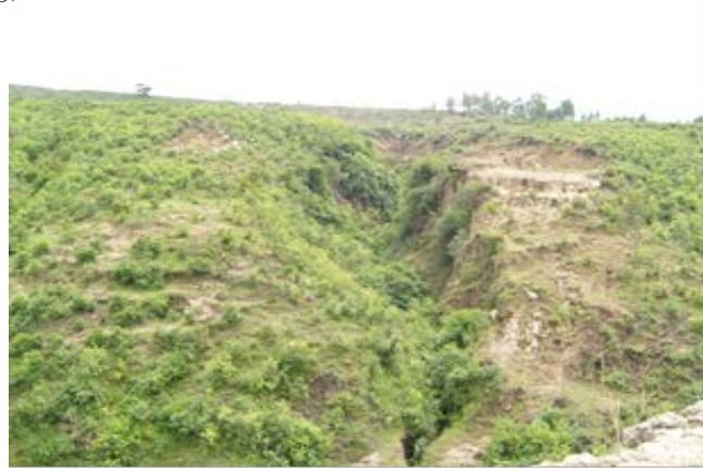
Deeply incised gully erosion following NW trending cracks
