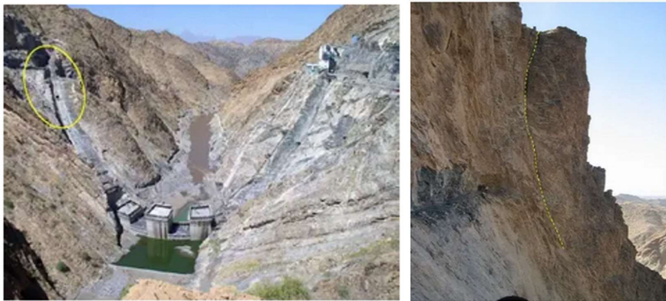
Figure 3: View of Tekeze dam site looking downstream; area of potential instability indicated in shape to the left and toppling condition, upper left abutment above dam to the right.
