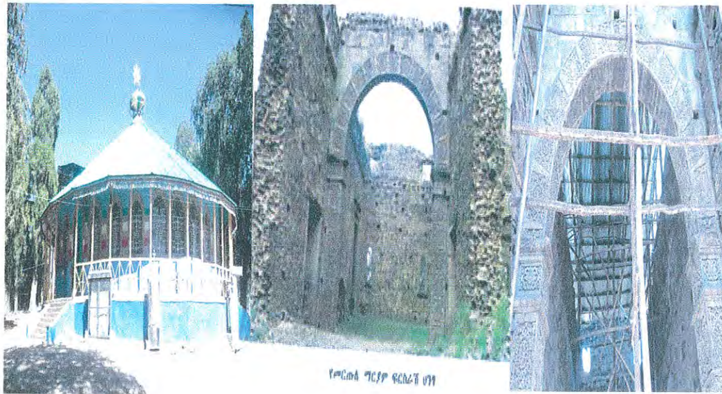
Figure 4.6 Mertu Le maryiam buildings, Source: ACTPDB, 2011 and field survey, 2014
