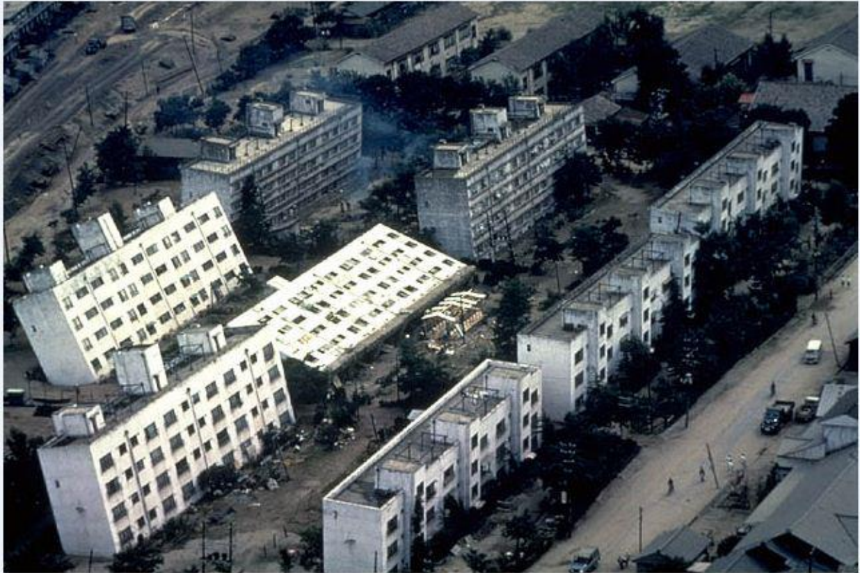
Fig. 2.7: Liquefaction induced bearing capacity failures of kawagishi-echo apartment buildings following the 1964 Niigata earthquake (courtesy of USGS)
