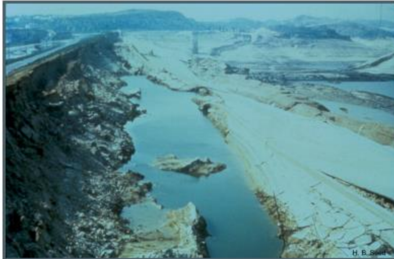
Fig. 2.8: Lower San Fernando Dam following failure of upstream slope in the 1971 San Fernando earthquake (Courtesy of EERC, University of California).
