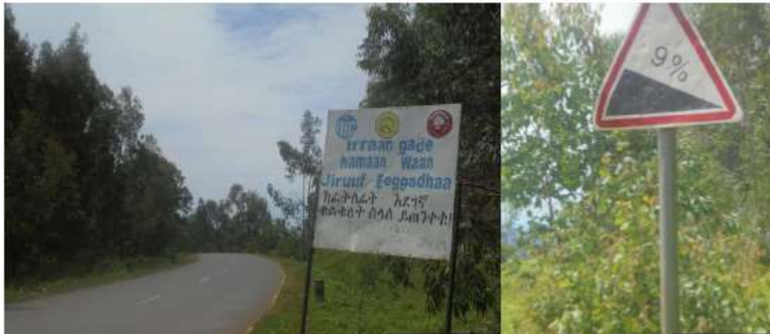
Figure: 4. 15 Warning posts at Qajela road section
