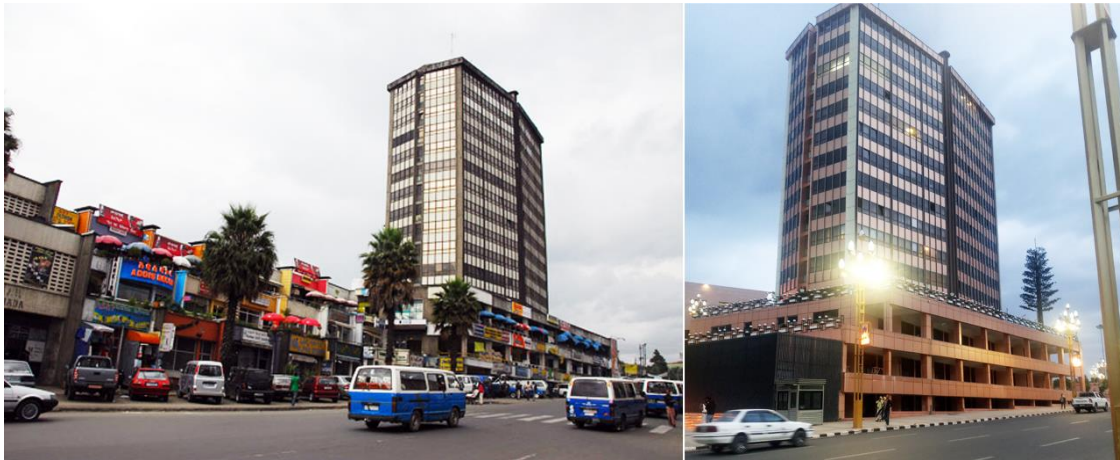
Figure 62: Arad building before and after the corridor development
