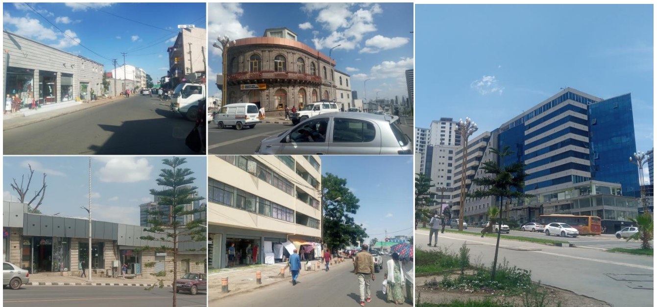
Figure 35: Some west facing buildings around the selected corridor segment
