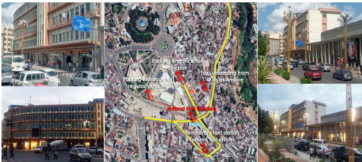
Figure 41: Site location and photos of case 1 'Mebrat Hail Building'
