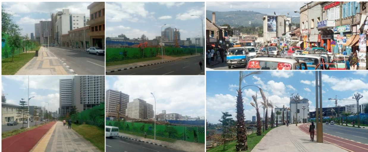
Figure 67: Reclaimed land behind Bbanko Diroma Building and road to Ras Mekonin Bridge
