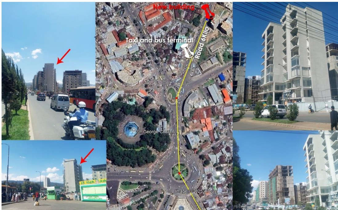
Figure 43: Site location and photos of case 3 ‘New building along the road to 6kilo’
