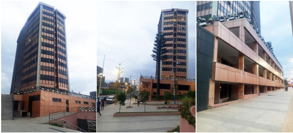
Figure 38: Arada building after the corridor development
