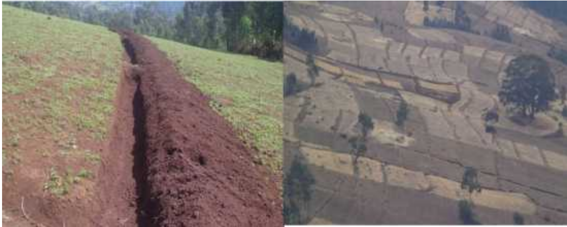
Figure: 5.3 Soil bunds Source: Field survey 2014
