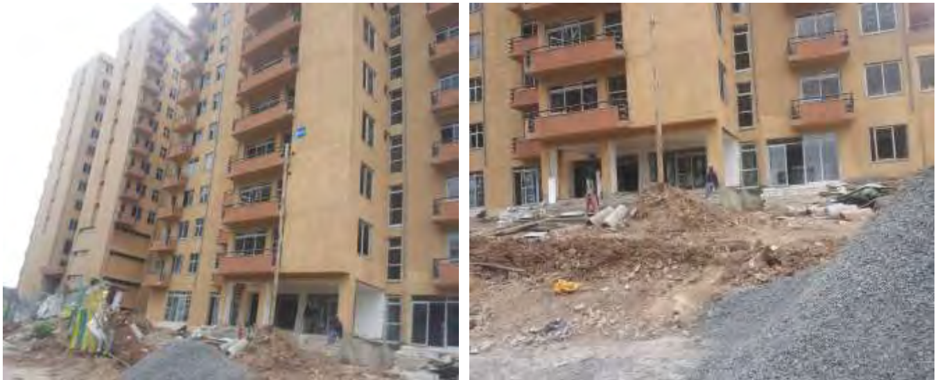
Figure 5. 2: Photos of Senga-Tera 40-60 housing construction projects (Taken on August, 2016)
