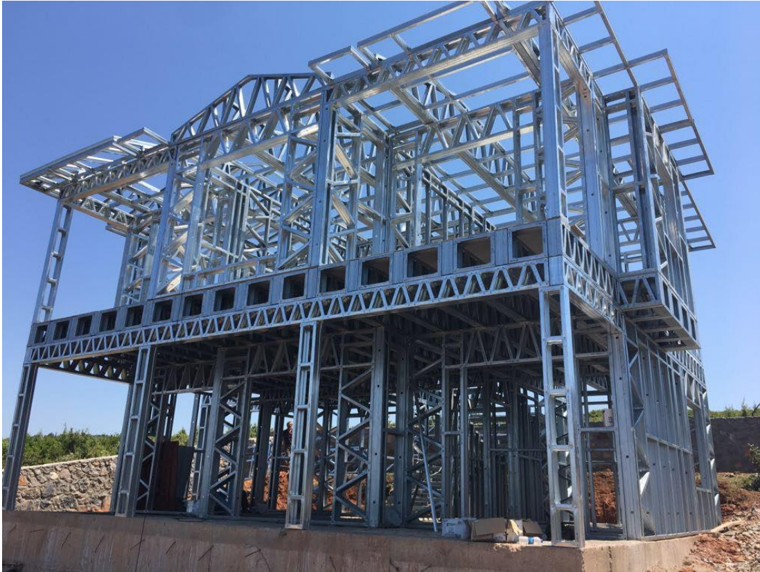
Figure 5: Pre-fabricated Housing Technologies
