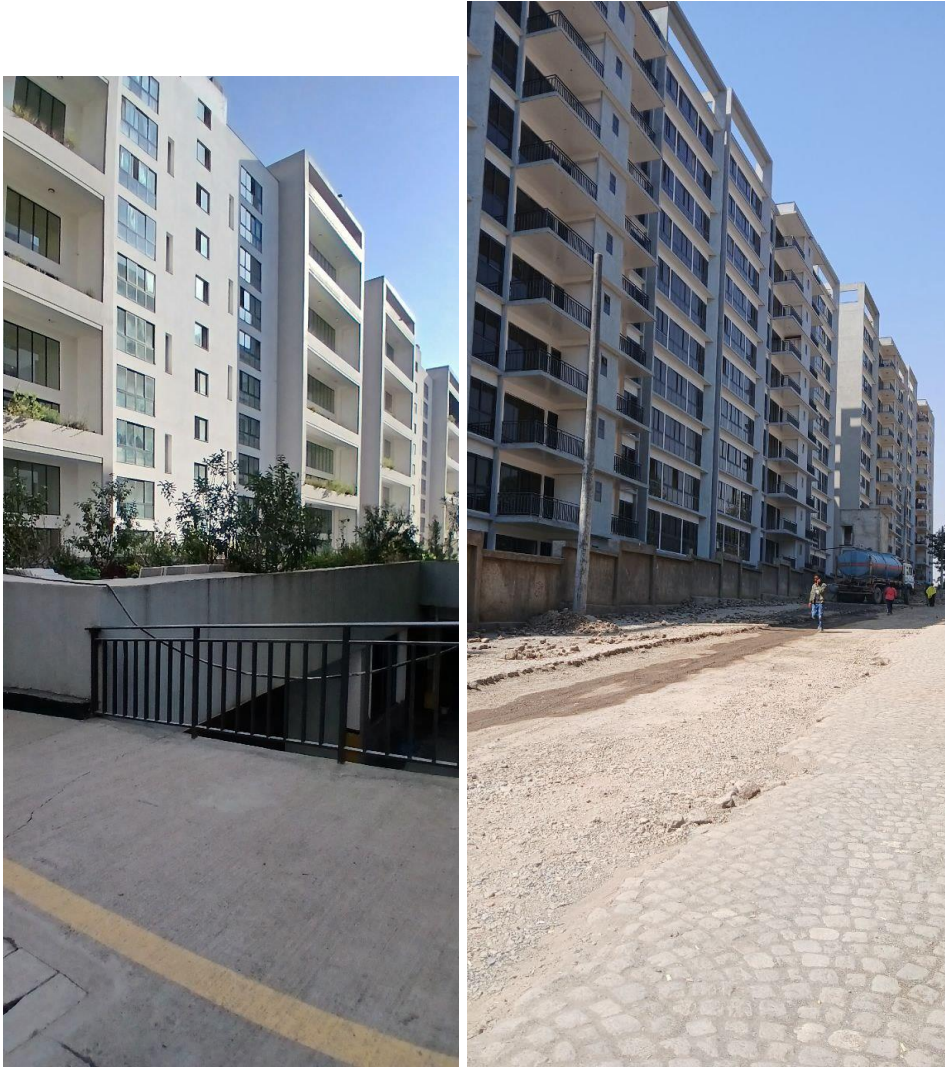
Figure 11: Houses built from Aluminum Form Work Technology Gerji site, Addis Ababa
