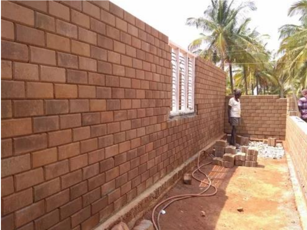
Figure 15: Mud Block house in construction Process
