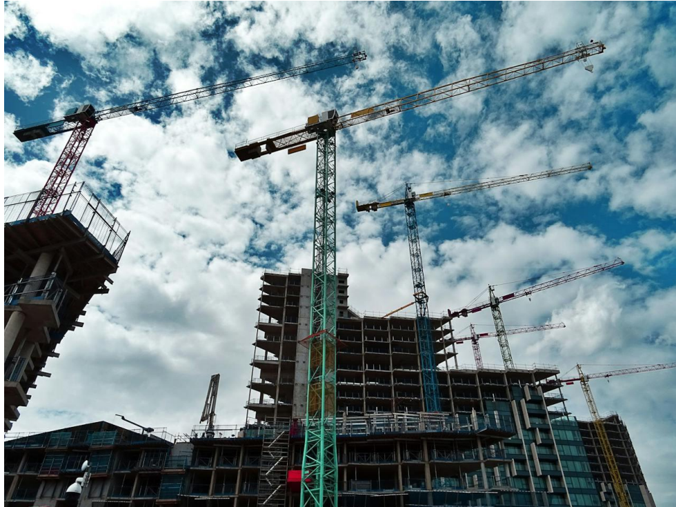
Figure 1 : Convention Housing construction
