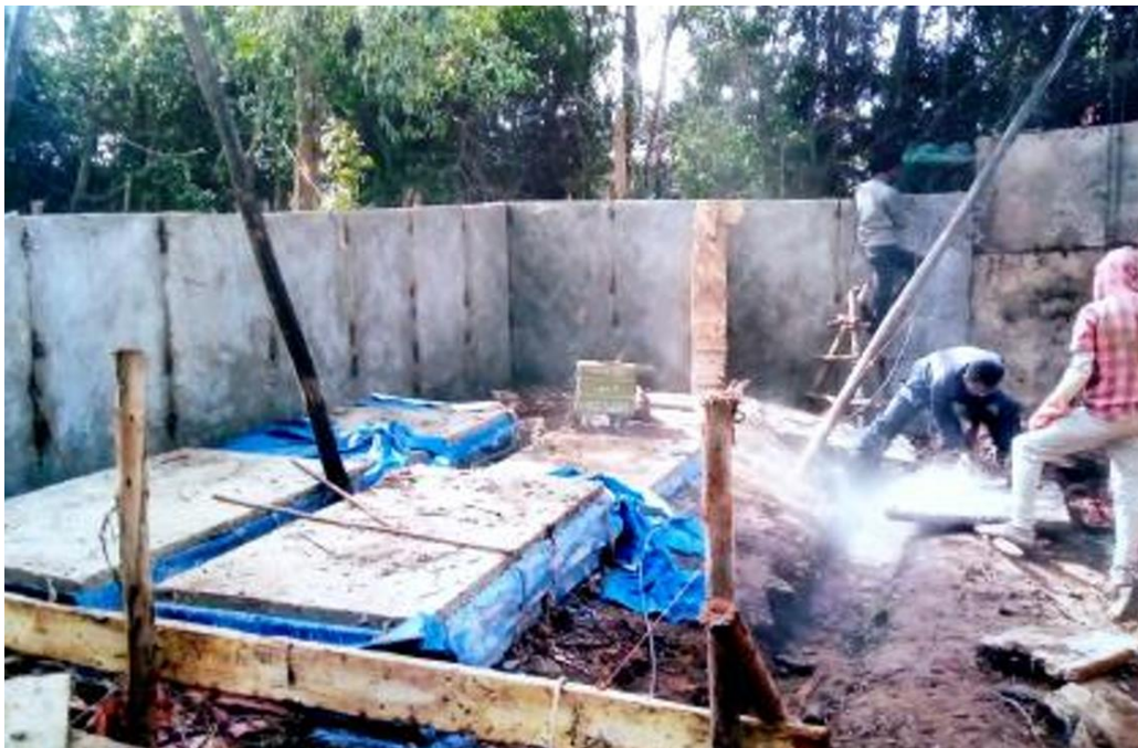
Figure 13: Middle of Building House with Qacha and Concrete
