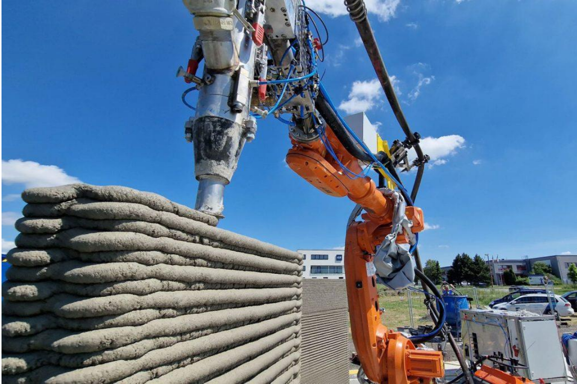
Figure 9: 3D printing on Process of building House
