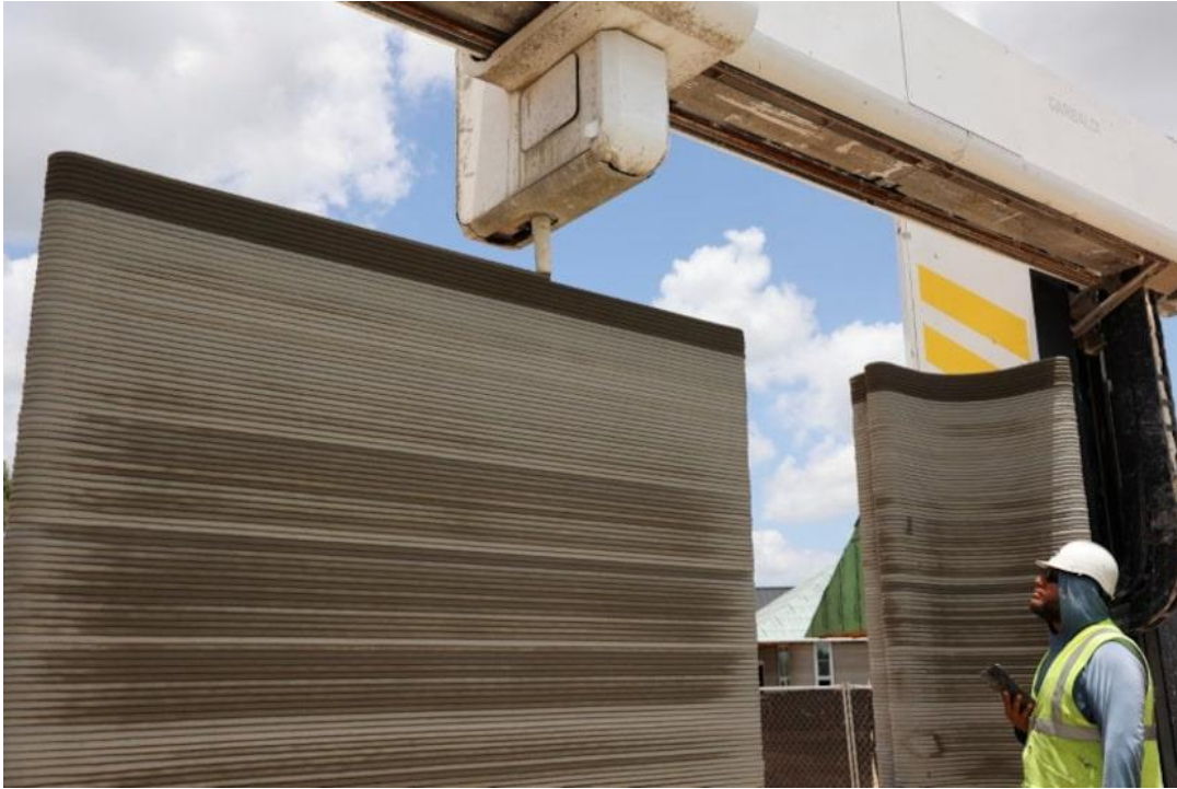
Figure 7 : 3D House printing Process
