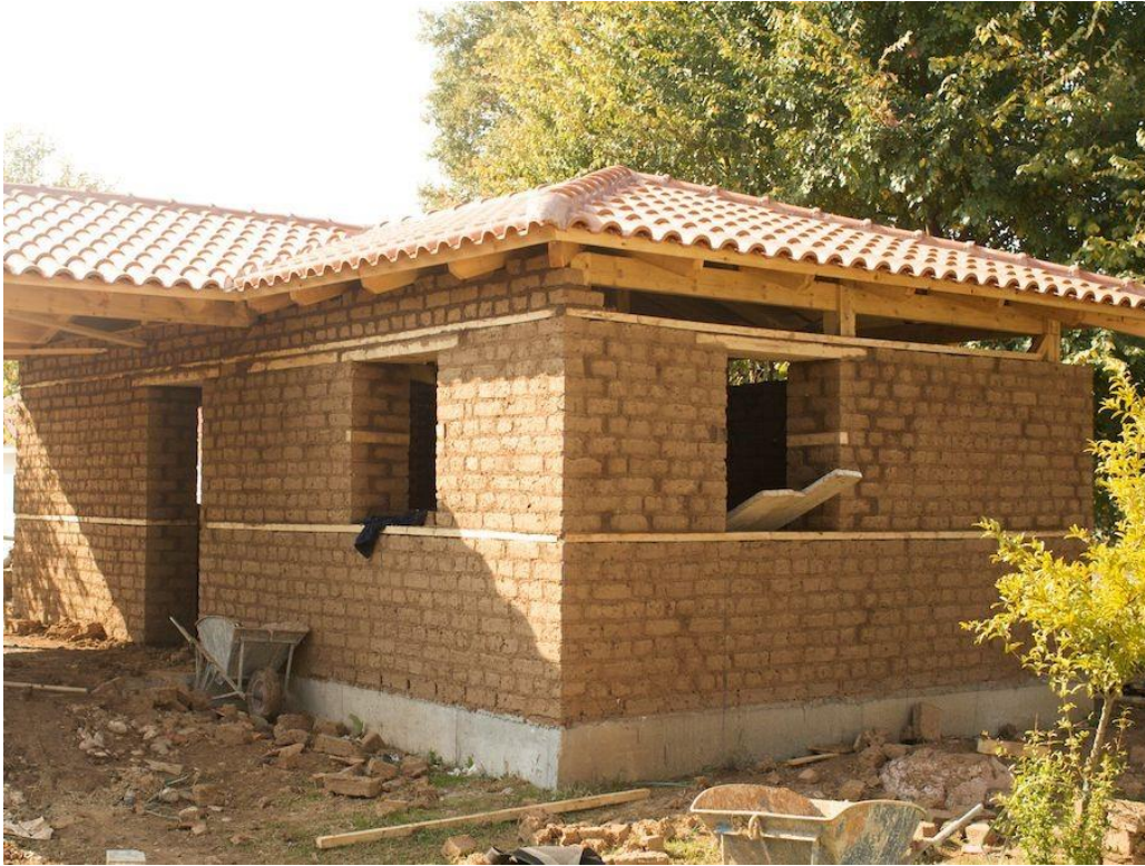
Figure 3: Mud Block Housing Construction
