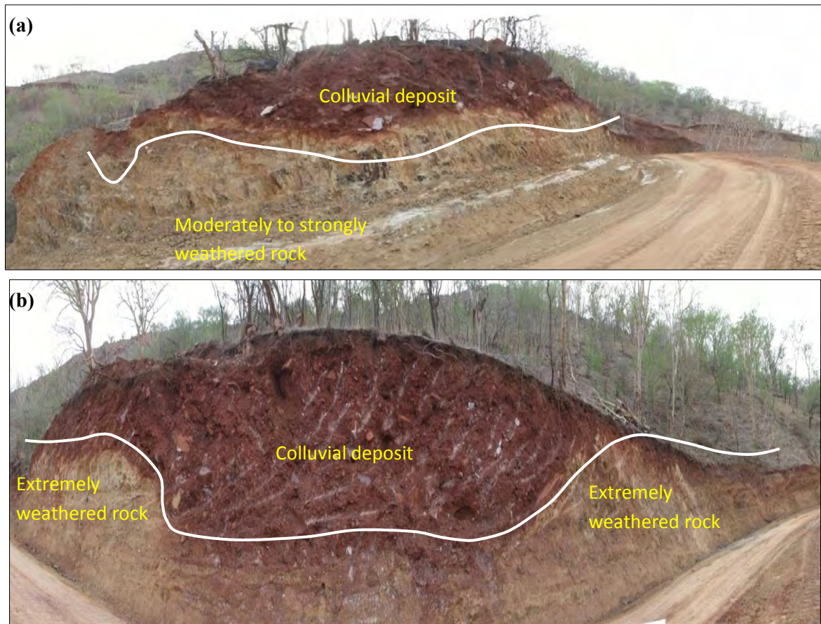
Plate 2.2: (a) and (b) Lateritic colluvial deposit as exposed along the access road cut. Note that the thicknesses of the colluvial deposits considerably vary from place to place.
