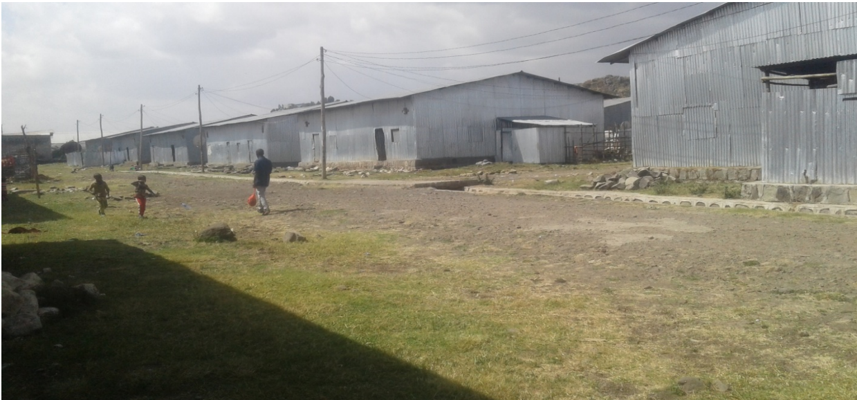
Figure 03: Picture of Sululta site corrugated iron made IDP shelters (Gelana site)
