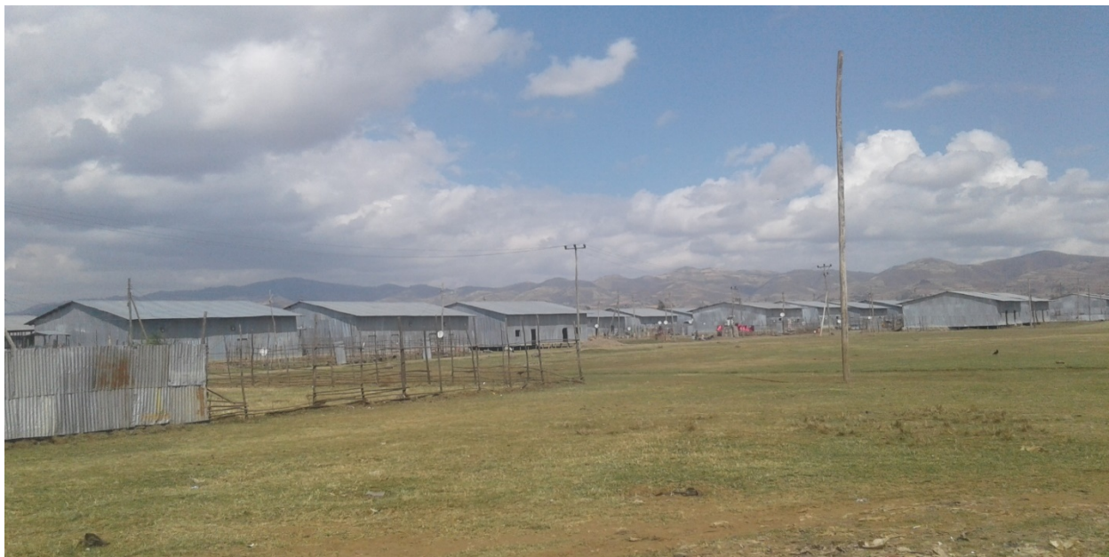
Figure 02: Picture of Sululta site corrugated iron made IDP shelters(Kajima site)
