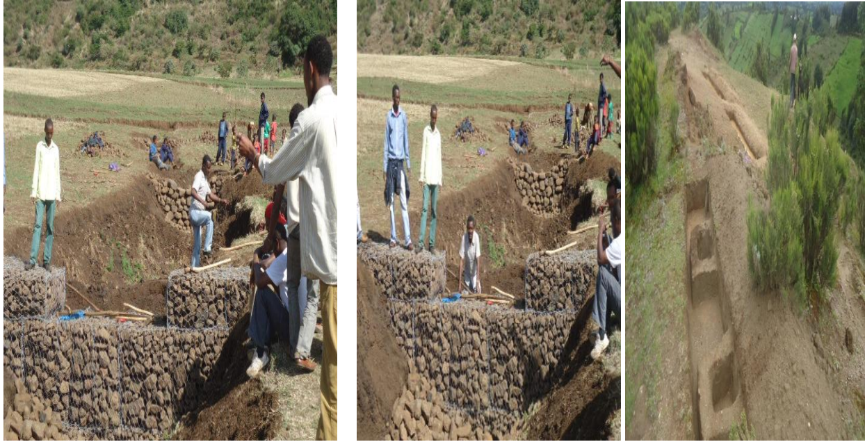
Figure 6. Some Environmental Conservation Activities Implemented Under SLM
