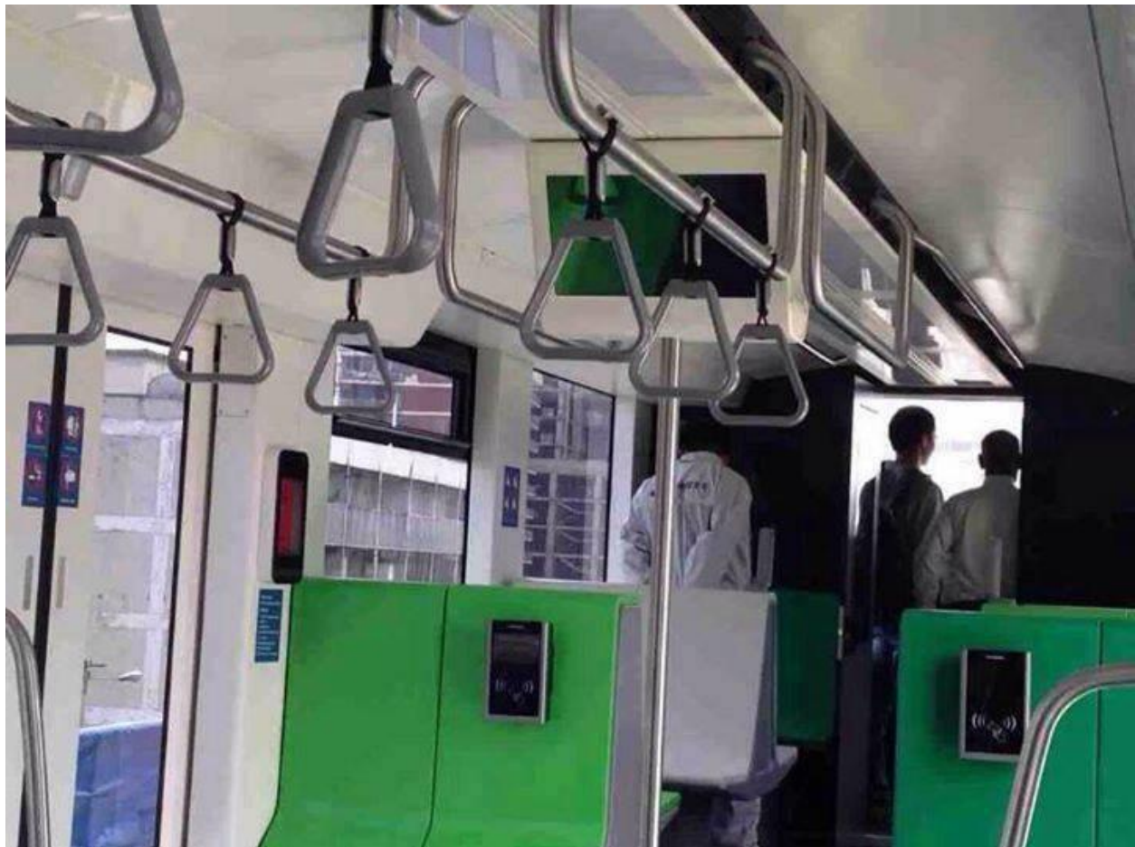
Figure 2-2: Smart Card Installed inside the Train
