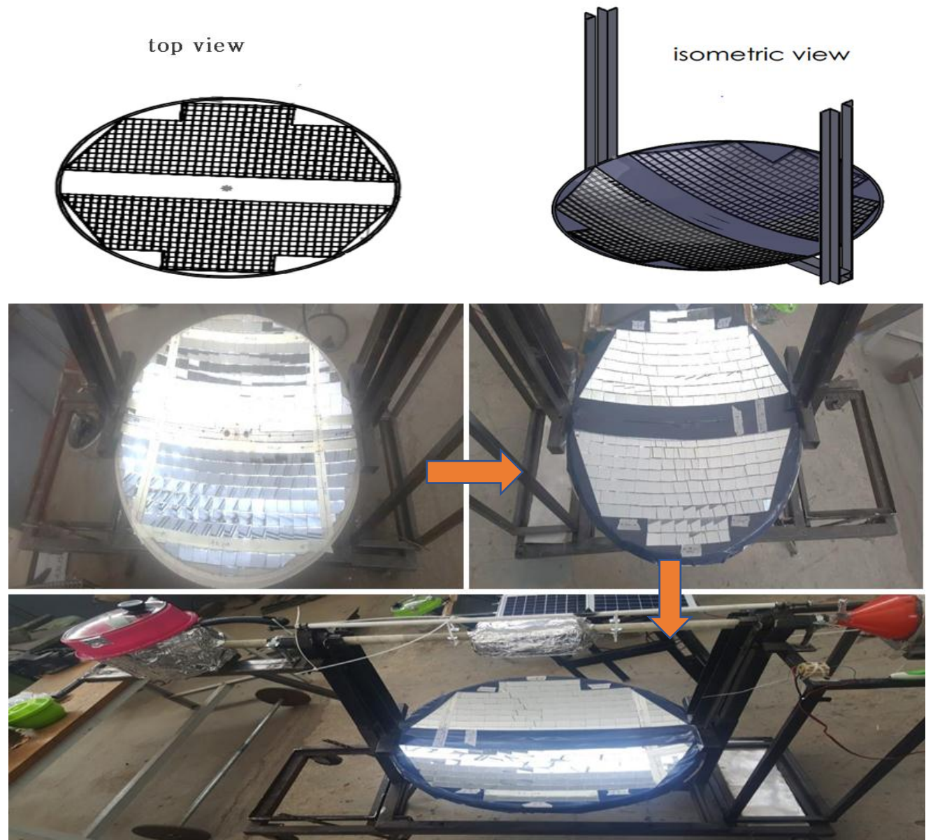
Figure 4-10: Assembly of the parabolic dish reflector to the dish support unit
