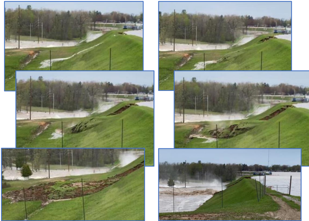
Figure 2. 5: Edenville Dam Developing to Full Breach Photo (ASDSO, 2020)
