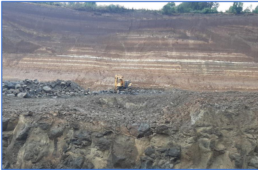
Figure 3. 7: Cutoff trench excavation of Fato dam during construction
