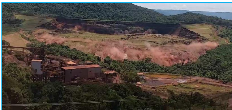
Figure 2. 4: Feijão Iron Ore Mine ("Dam I") Breaching Photo (ASDSO, 2020)
