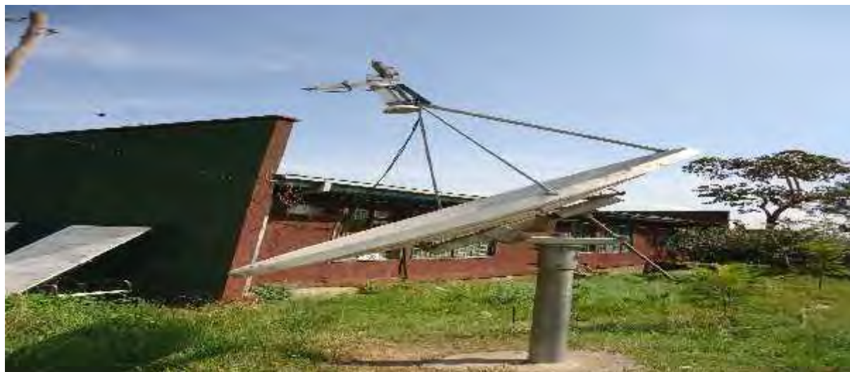
Photo 1: VSAT antenna equipped in a school in rural area in Ethiopia
