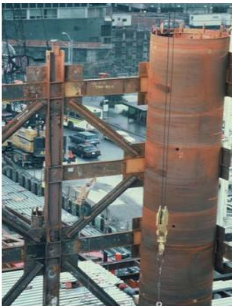
Fig. 4: Concrete filled tubular steel-concrete composite column during construction [Roberto et al. (2013)]
