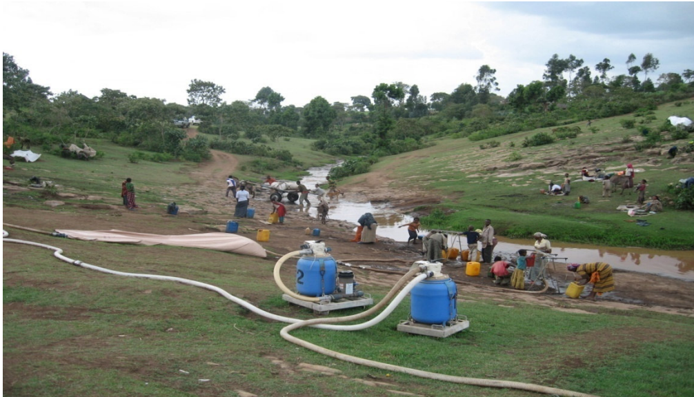
Figure 9.2.3: EMWAT kit supplied by UNICEF for water treatment positioned at the source so as to benefit as many people near to Kassa CTC site, Shashamane, July 2009
