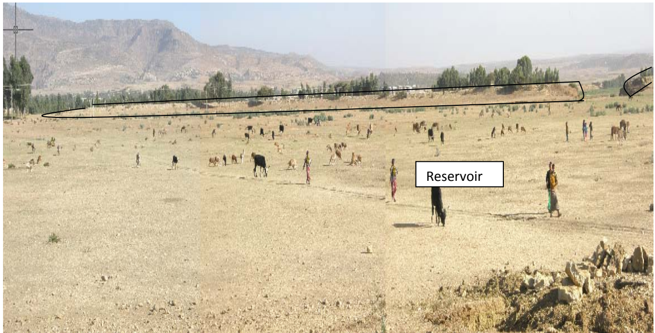
Figure 1.2 General view of Hizaeti Afras dam site.
