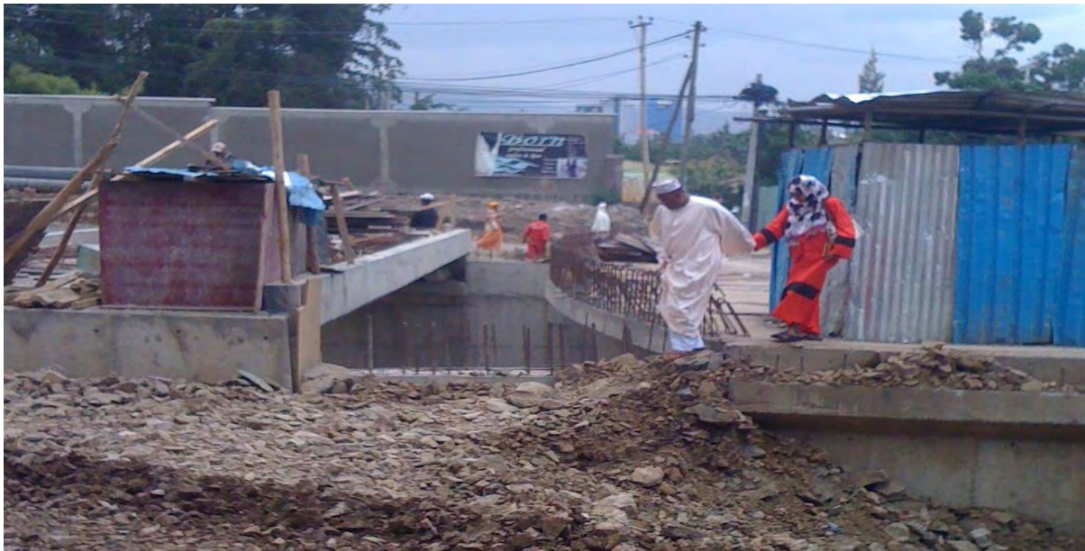
Figure 5.1 Road construction in Addis Ababa
