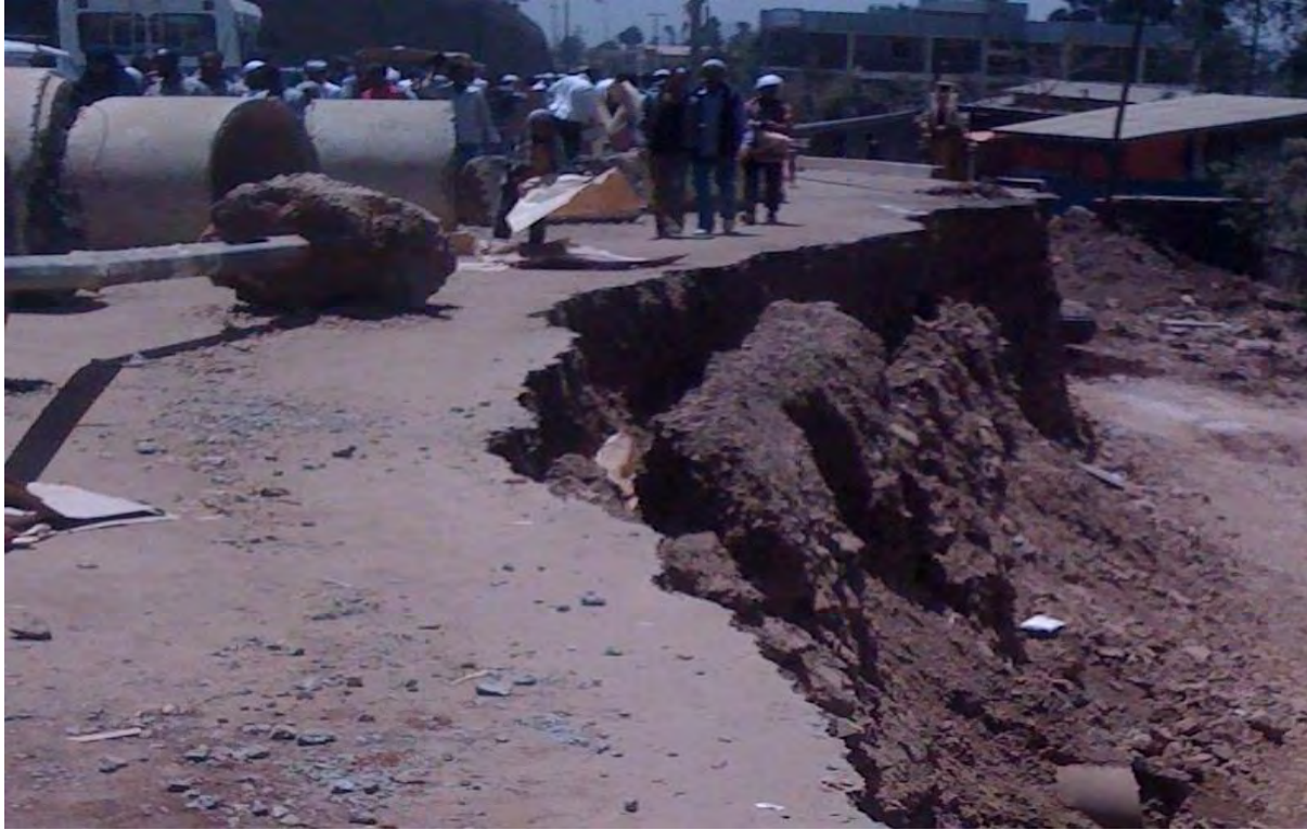
Figure 5.3 Road construction in Addis Ababa
