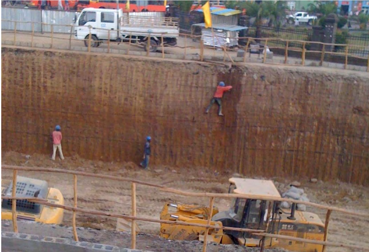
Figure 5.4 Railway construction in Addis Ababa
