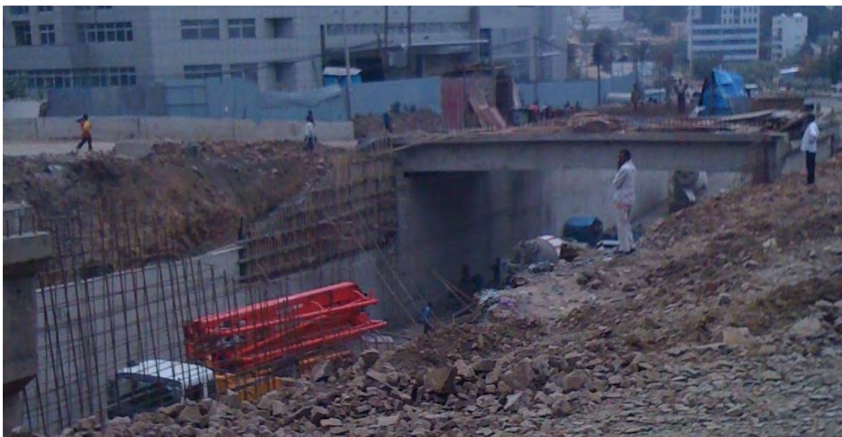
Figure 5.2 Road construction in Addis Ababa
