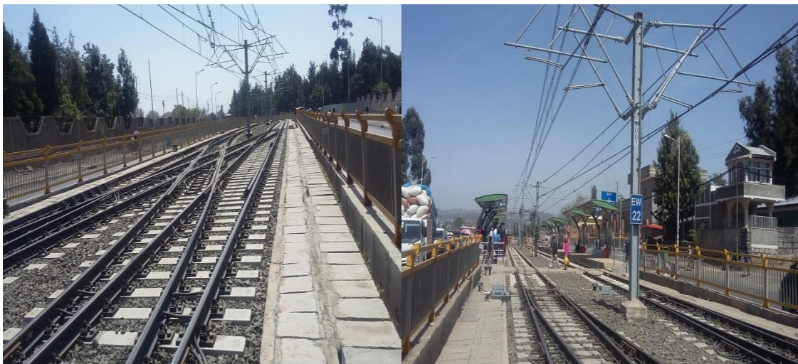
Figure F-5: AA-LRT Elevated Track Pictures around at Estephanos
