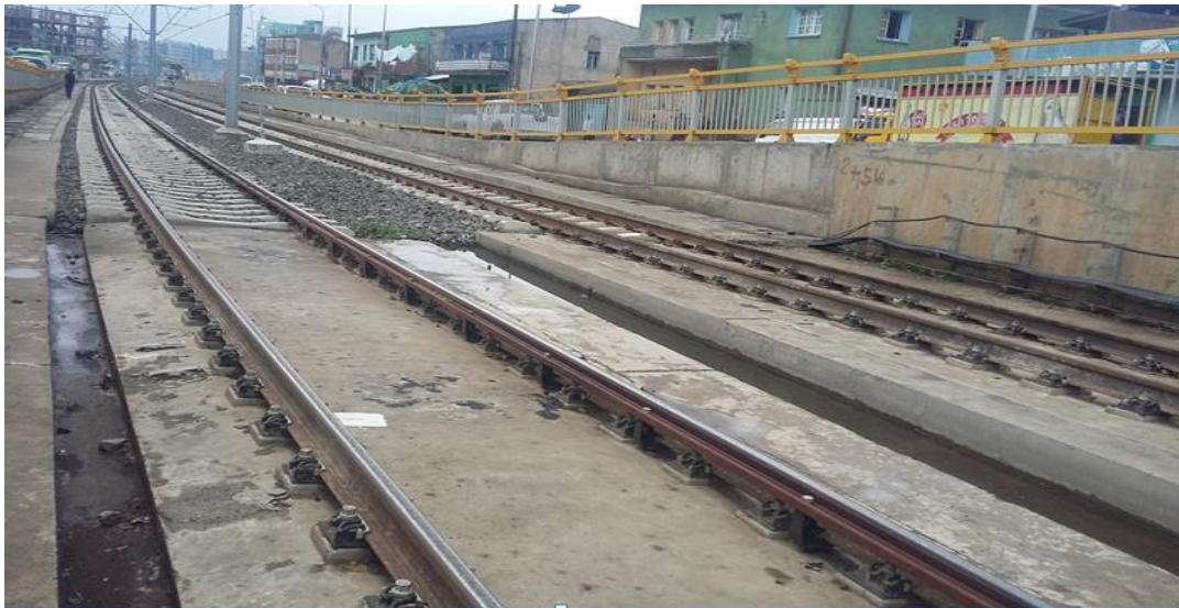
Figure 4-2: Slab track at transition section AA-LRT project
