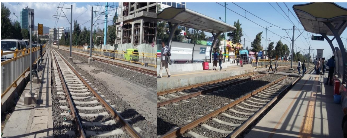
Figure F-11: AA-LRT Track Pictures around at Mesholekia
