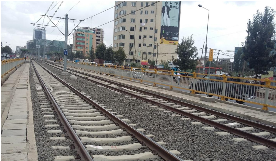
Figure 4-1: Ballasted track at grade/ground section AA-LRT project
