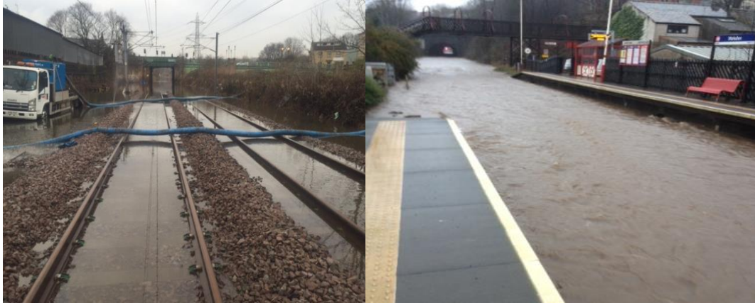
Figure 2-4: Flood problems on railway track
