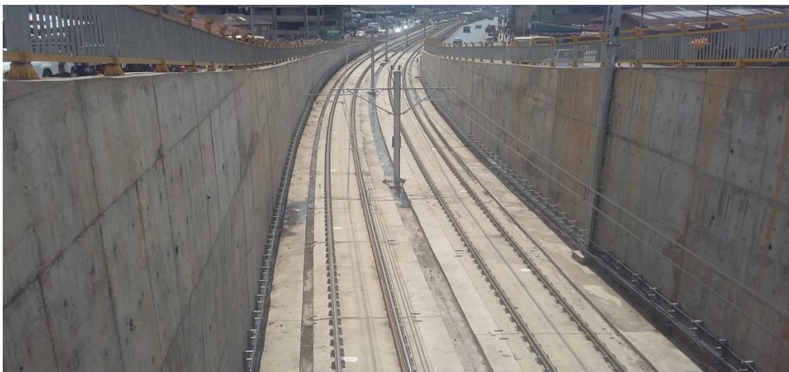
Figure 3-5: AA-LRT Transition Section Track Picture at Atikilt tera
