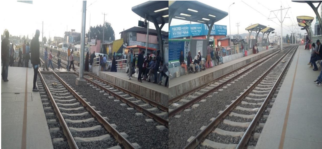
Figure F-9: AA-LRT Track Picture at Gojam Berenda
