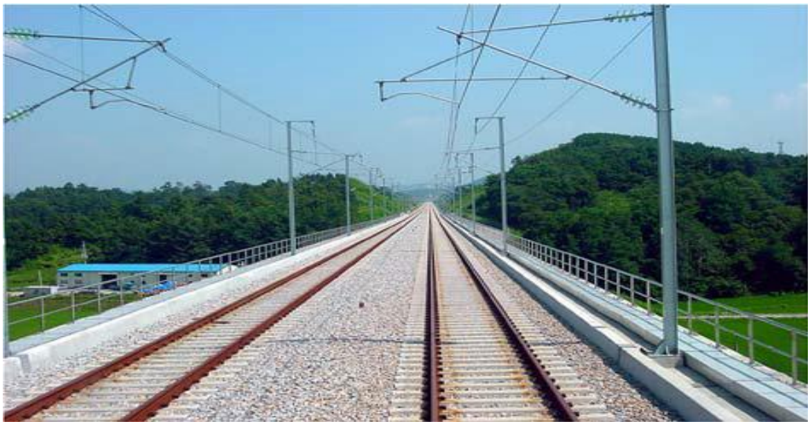
Figure 2-1: Ballasted HSL track of KORAIL (Esveld, 2010)
