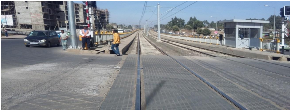
Figure 3-3: AA-LRT Track Level Crossing Picture around CMC
