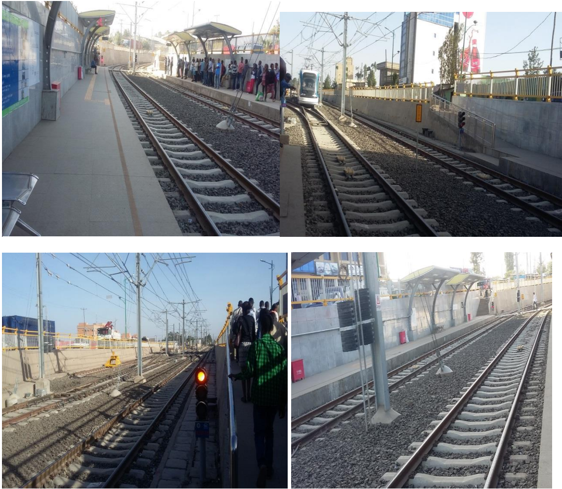
Figure F-15: AA-LRT Track Pictures around at Kalit
