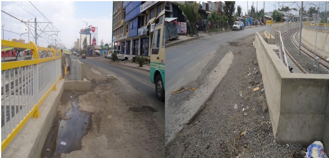
Figure 3-6: AA-LRT Track Picture around at Kality
