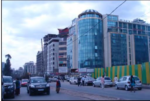
Pic - 3.7: Usage of parking spaces and problems.
