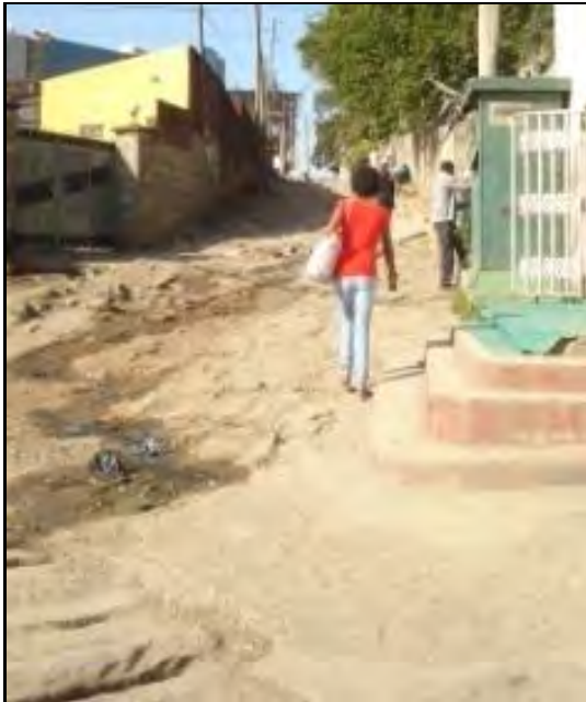
Pic - 3.124: Existing poor Street condition.
