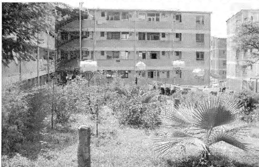
Figure 8: Water storage in Mikililand condominium sites of Kolfe keranio Addis Ababa
