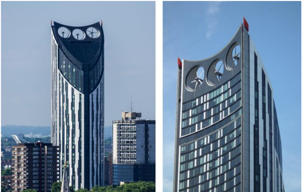
Figure 2.10: Building integrated wind turbines with horizontal axis (Strata SE 1, London). (Dymock & Dance, 2013)
