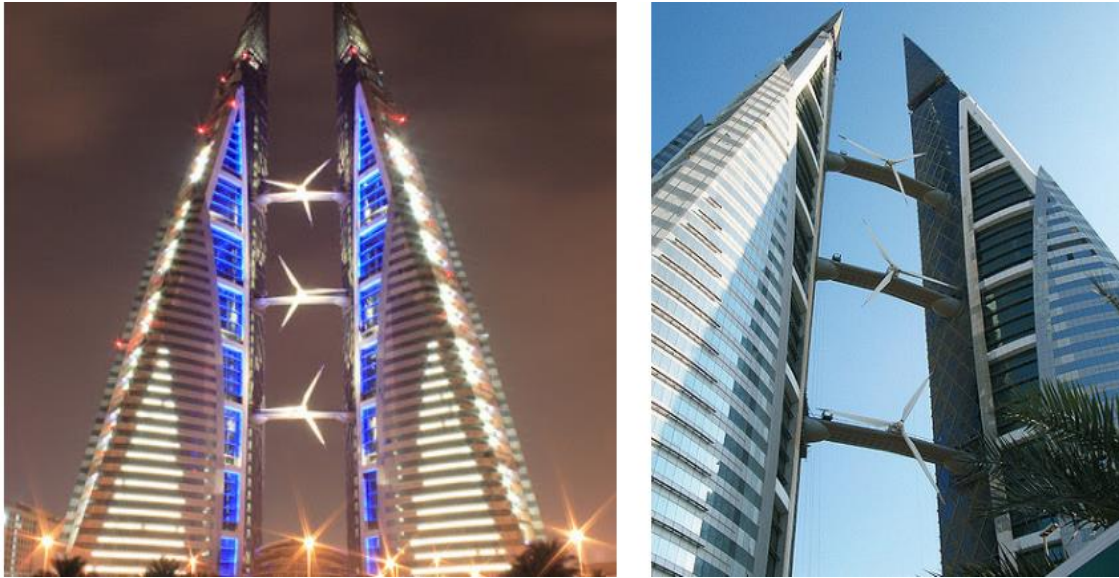
Figure 2.11: Building augmented wind turbine, horizontal axis (World Trade Center, Bahrain). (Haase & Löffström, 2015)
