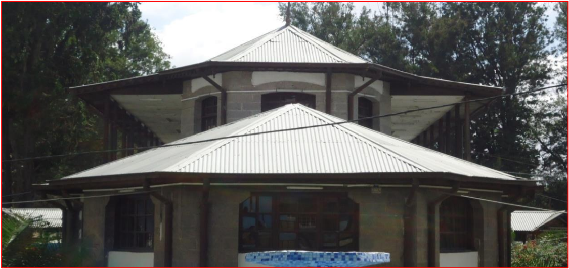
Figure 4.13: Picture of Bete Saida hospital building
