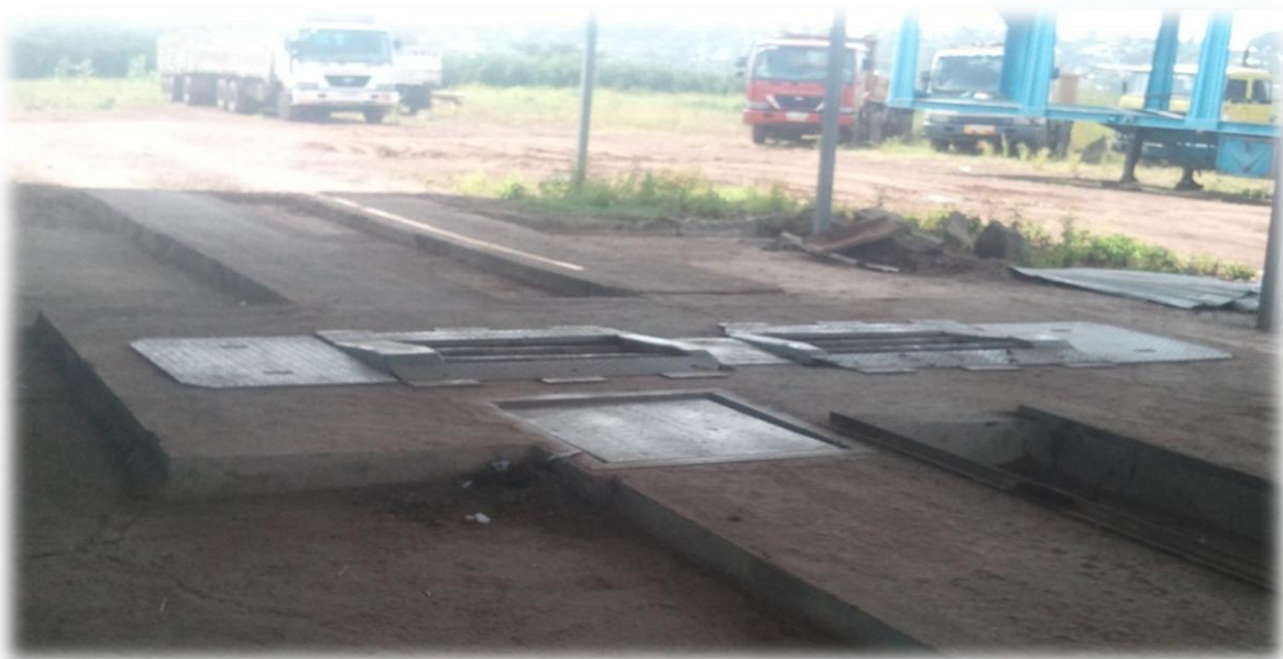
Figure 3.2: Vehicle Inspection Pit
