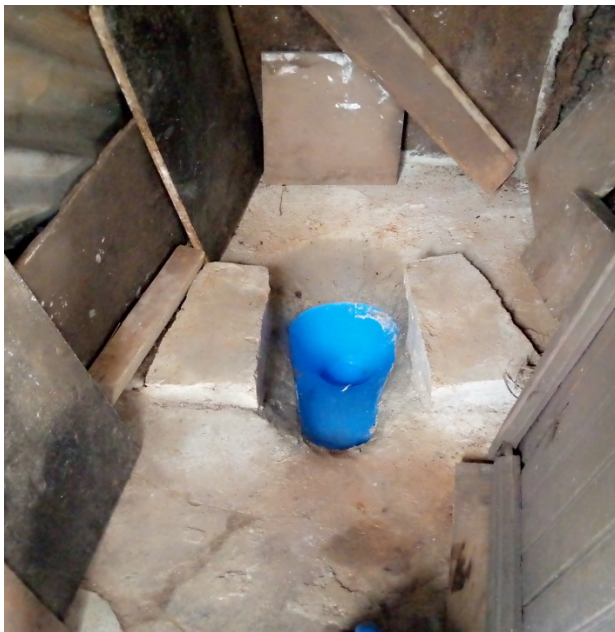
Fig. 4.1. Installed SATO toilet set
