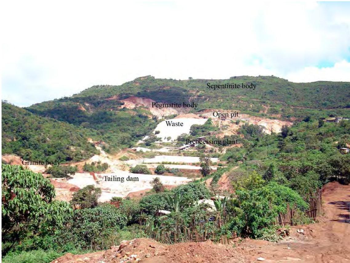
Figure 5. 13. Kenticha Tantalum deposit with location of open pit, processing plant, waste dump and tailing dam.
