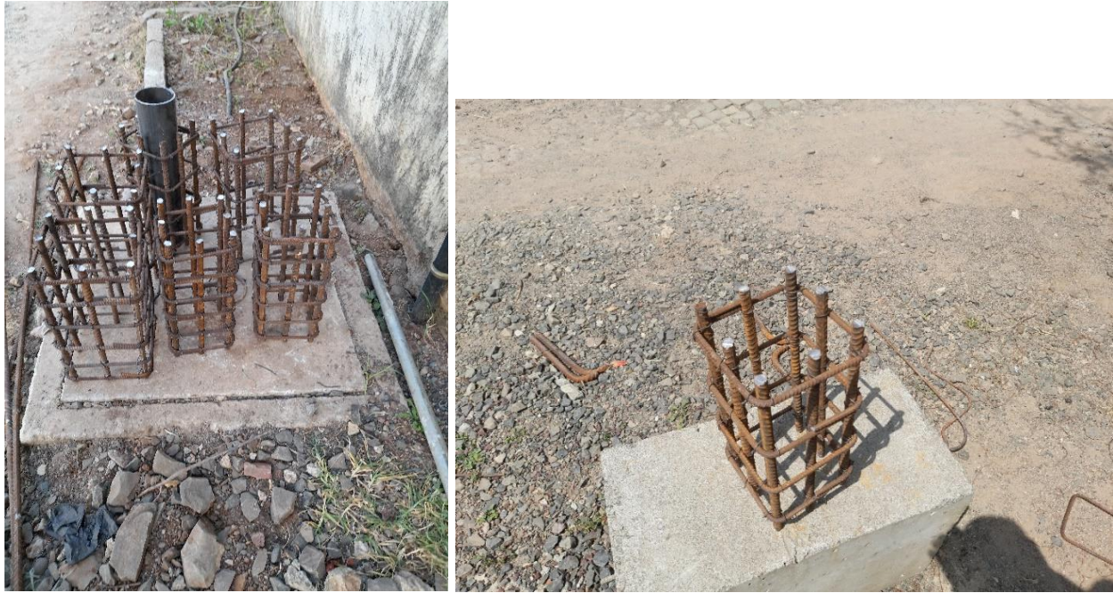
Fig 3. 4 reinforcement preparation
