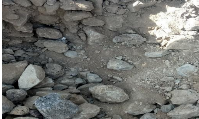
Figure 3-5 Fouling Materials on the track
