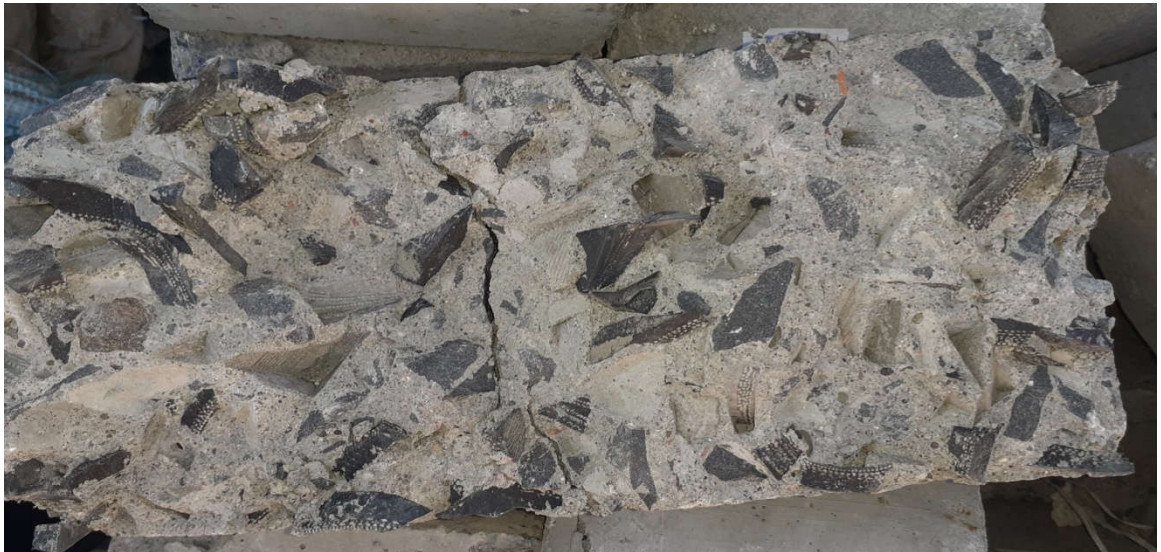
Rubber particles distribution in concrete matrix after failure with tensile loading
