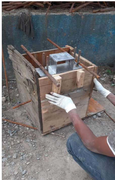
Preparation of form work to cast the clamping system
