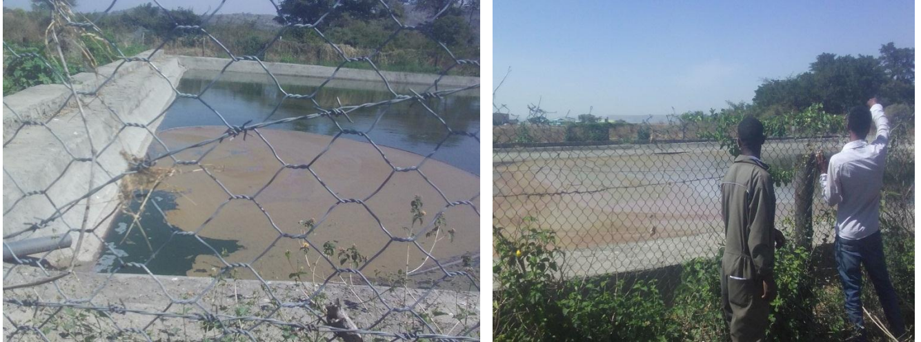
Figure 10 This is evaporation pond build by Castel Winery at the back of their wine yard. Residue from the factory is transported through pipe and collected in this pond.
